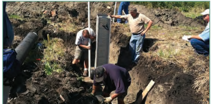
A bioreactor is being installed to remove nitrate from tile water.
